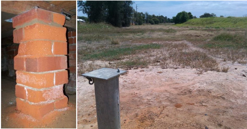
Figure 1: Salt damage to footings (left) and salt scalding (right), Turvey Park, Wagga Wagga.
