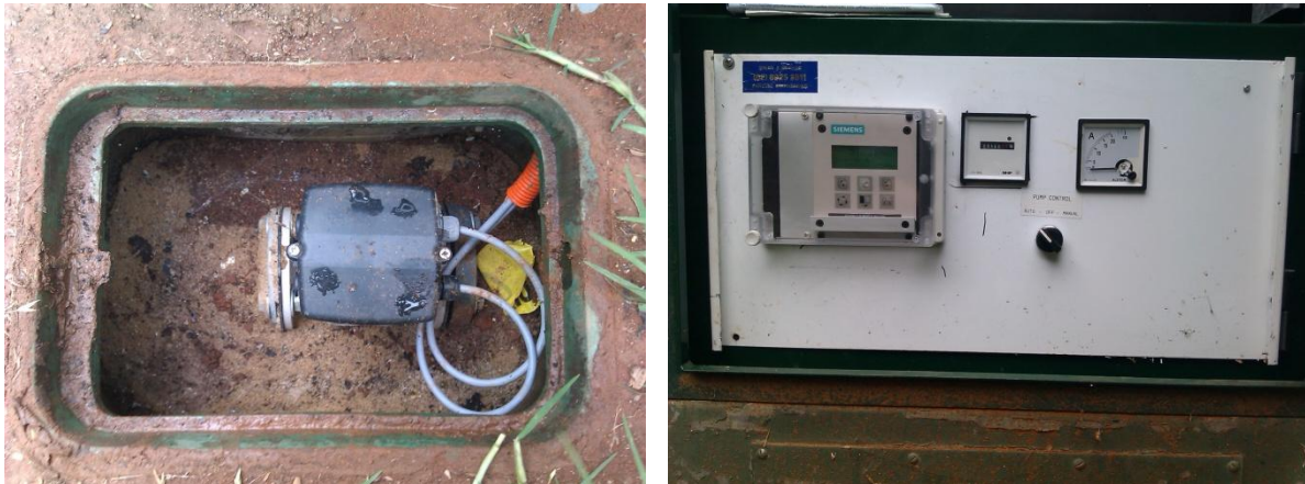
Figure 7: Electromagnetic flow meter and transmitter fitted to six Calvary Borefield pumps.
