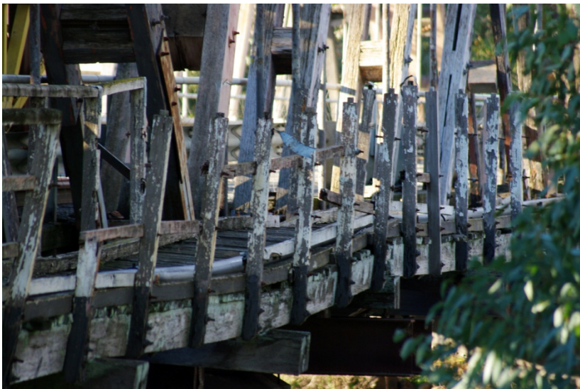
Figure 4-5: Handrail along span 1
