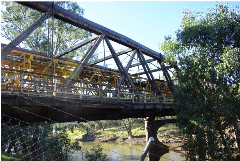
Figure 4-1: Span 1, with the yellow steel stabilisation truss
