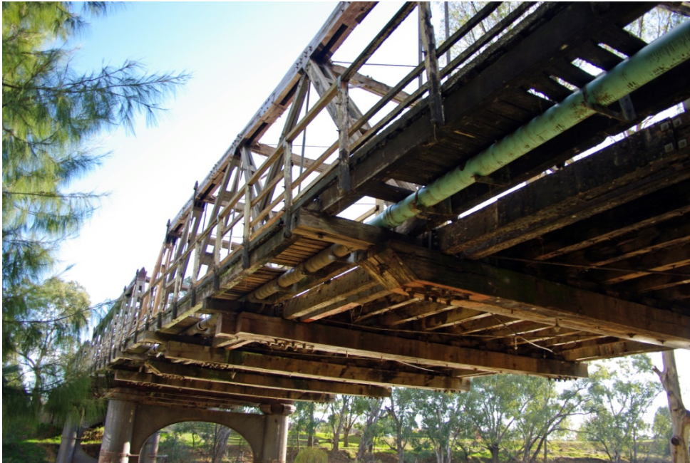
Figure 4-4: Missing parts of the walkway can be clearly seen
