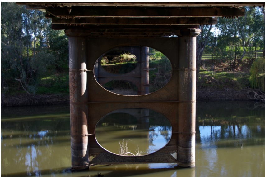
Figure 4-9: River piers, viewed from the eastern abutment
