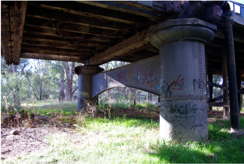
Figure 4-10: In ground pier on the western side
