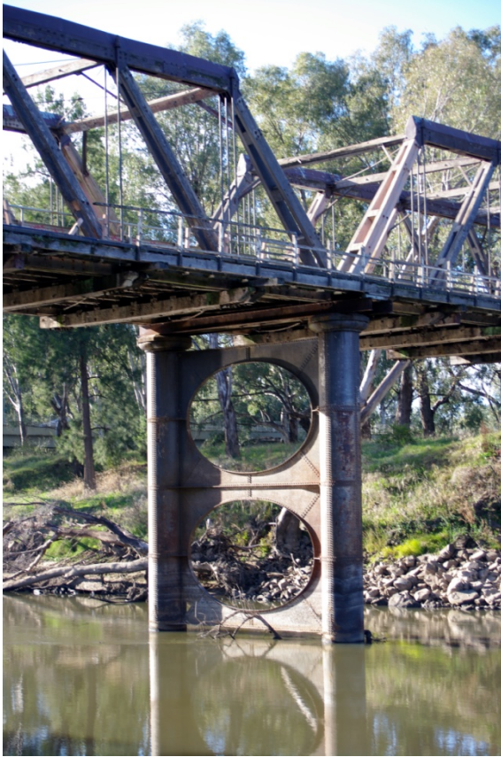
Figure 4-8: Eastern steel pier
