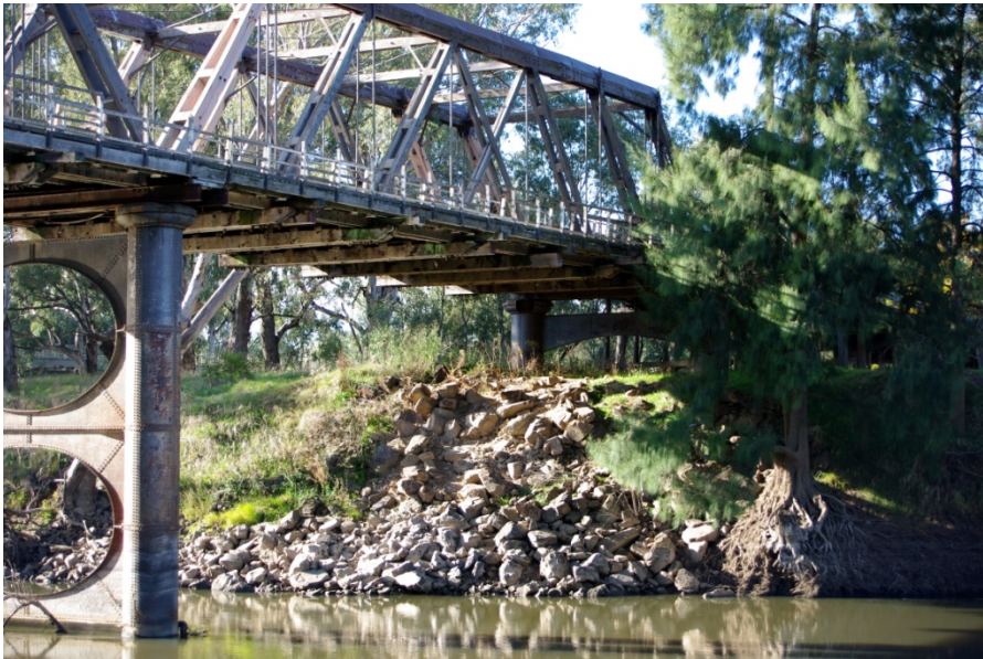
Figure 4-6: The Eastern abutment is reinforced with rough laid rocks
