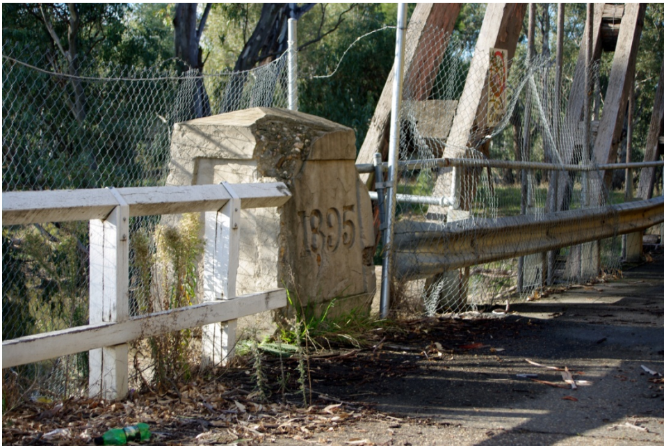
Figure 4-15: Date plaque commemorating the year the bridge was built, although it is unknown if this forms part of the original fabric of the bridge.
