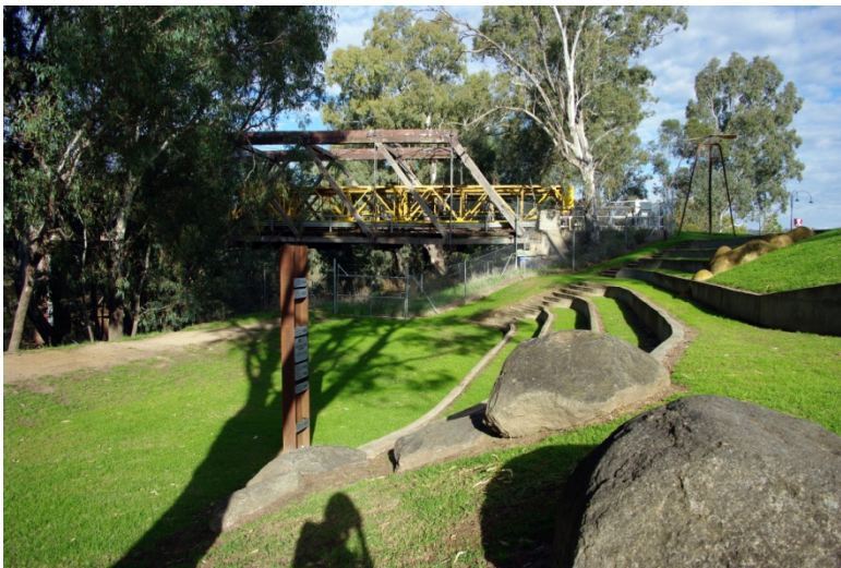
Figure 4-16: Sculpture park, amphitheatre and the western side of the bridge
