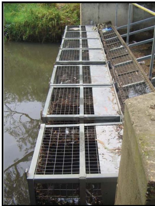
Plate 2: Photograph displaying the gross stormwater pollution traps at the inflow to the Lagoon from the western end.
