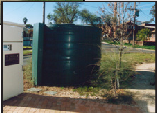
Right: Pump and storage tank at Emblen Park
