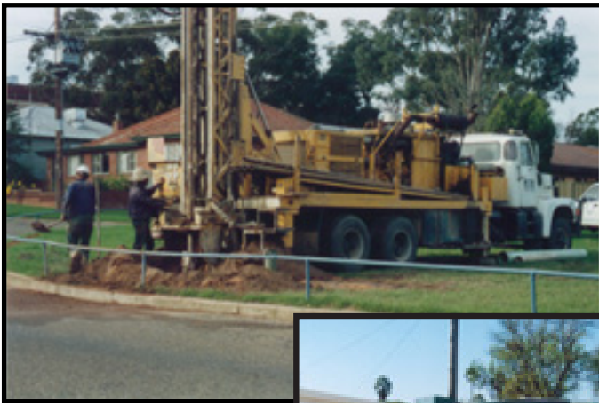
Left: drilling a de-watering bore at Emblen Park in 1999
