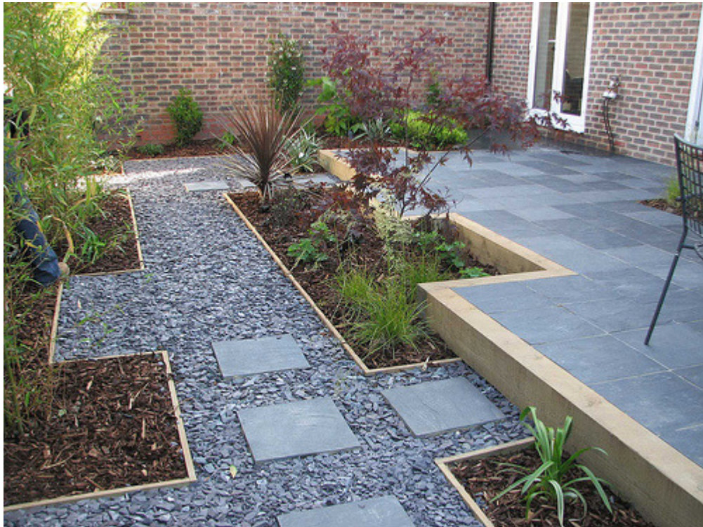
Figure 1: Garden includes blue slate pavers, crushed blue slate, mulched garden beds, low water use native plants and grasses, timber edging
