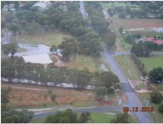
Photo 60: Plumpton Rd/ Nelson Rd/ Springvale Dr intersection
