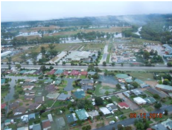
Photo 9: Moorong St/ Flowerdale Rd intersection
