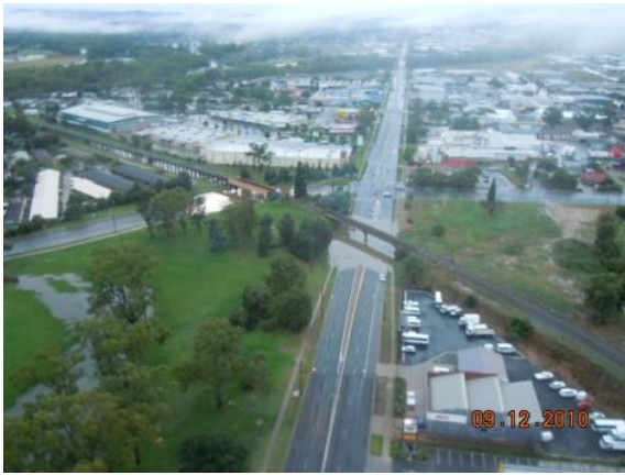
Photo 48: Bolton Park to the left and low points on Tarcutta St and Sturt Hwy under Railway.
