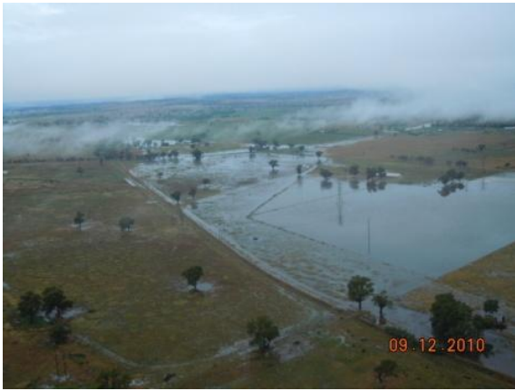
Photo 54: Inundation behind railway embankment (between Marshalls Ck and Koorringal Rd,
