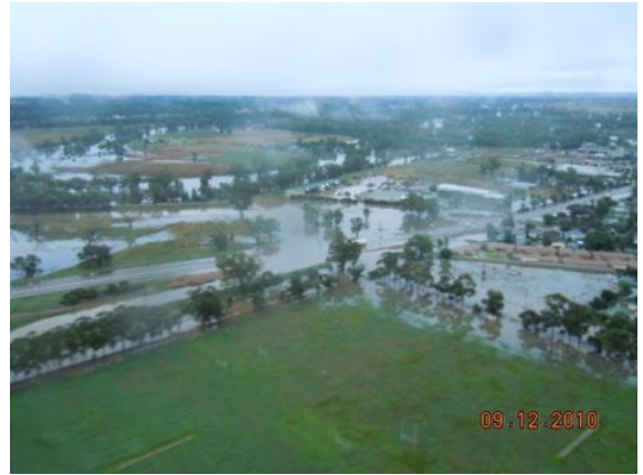
Photo 4: Edward St/ Morrong St intersection (2)
