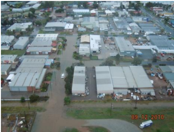
Photo 43: Nagle St looking west
