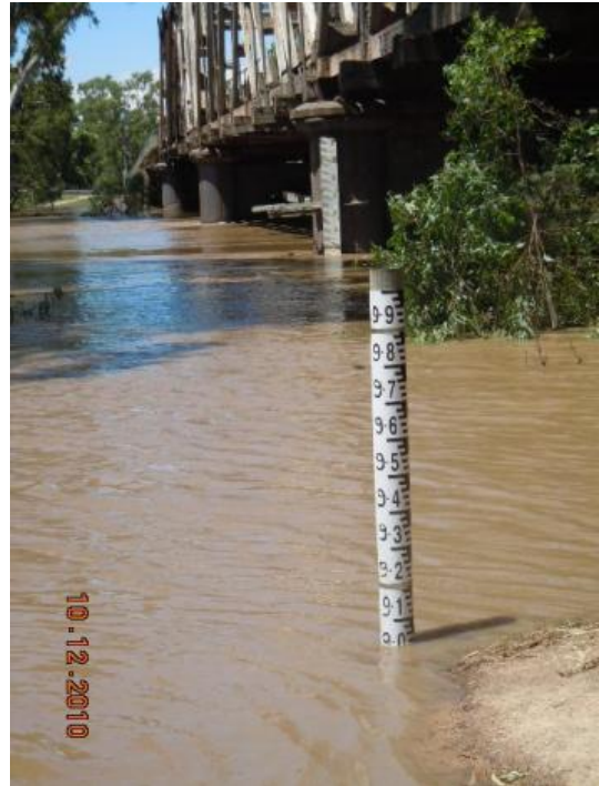
Photo 76: Hampton Bridge gauge
