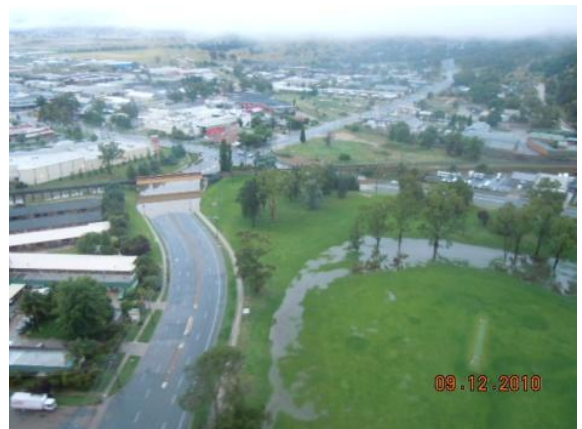
Photo 47: Bolton Park and Tarcutta St underpass
