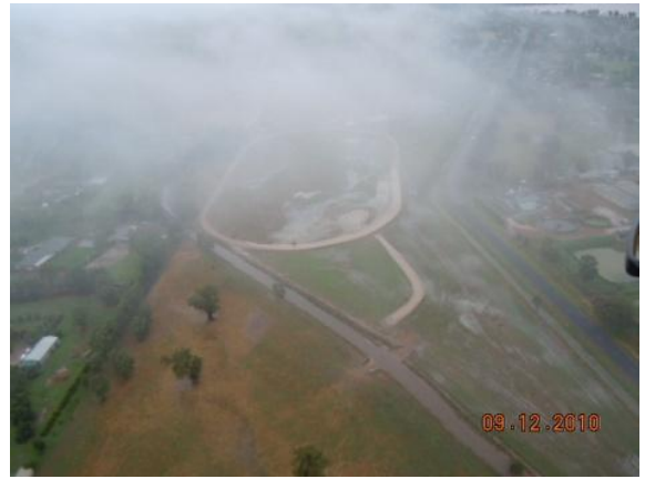
Photo 57: Crooked Ck/ Sycamore Drain upstream of Vincent Rd.
