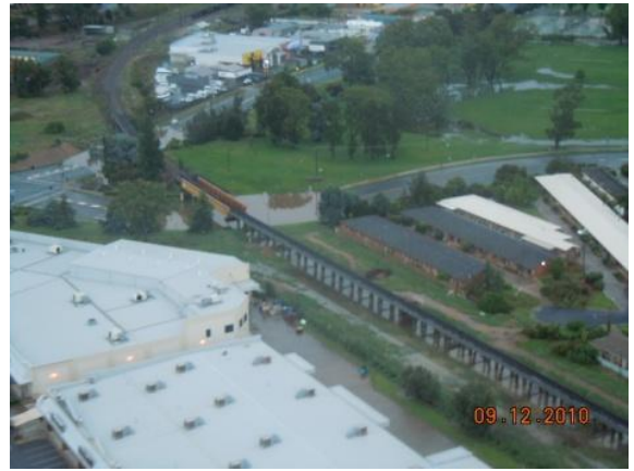
Photo 45: Railway underpass on Tarcutta St
