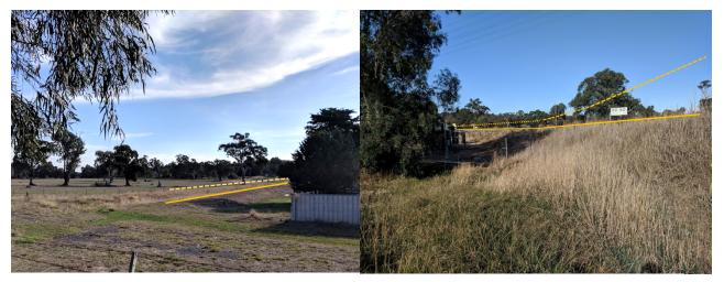
East end (left) and west end (right) of levee with crest in yellow and approximate additional height in yellow
