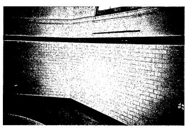
The octagonal bath house is constructed of granite blocks. The sunken bath and walls to approximately head height are tiled and the ceiling is of pressed metal. The bath house is situated near the lake. The level of the lake was raised some years ago, and it now almost laps at the base of the building. As a consequence of this the building has begun to deteriorate rapidly; major cracking has appeared in the floor and walls and the pressed metal ceiling is rusting out.
