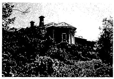
Big Springs homestead, east elevation. This elevation has been modernised during the late 20th century. The bay window, which was previously identical to the one below [south elevation] was altered and the verandah was removed and replaced with a pergola.
