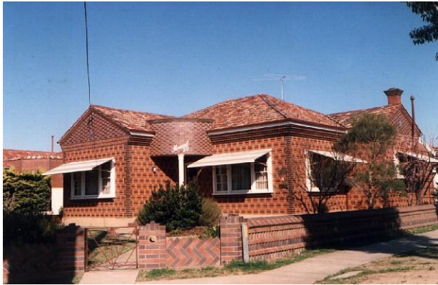
20 Docker Street, polychrome brickwork, built for Mr Willis of Willis Bricks
