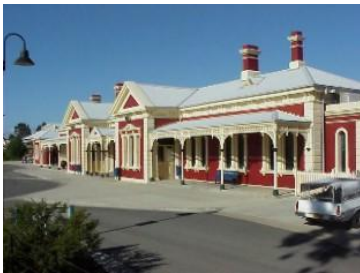
Wagga Railway Station [1879]
