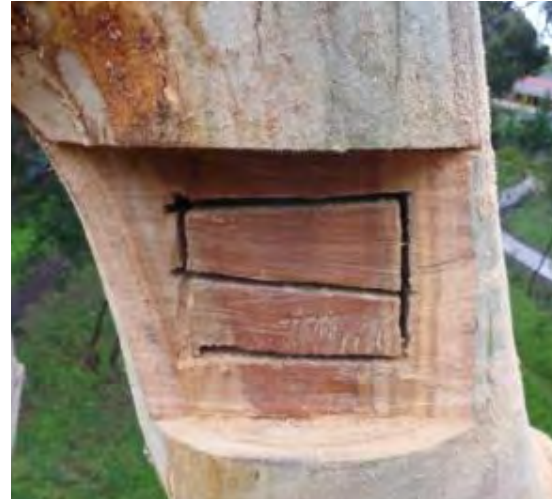
Figure 8: Horizontal boring cuts
