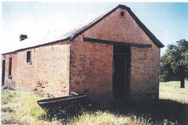
The Coach House, note the formerly much wider opening which has been bricked up to form a standard doorway, and the weathering of the soft bricks. Both sections of the building are subject to rising damp and windows have rotted out.
