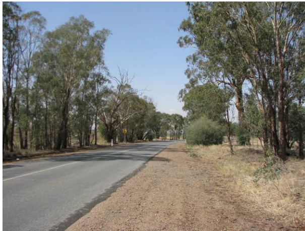
Photo 1: Looking south along western edge of road.
