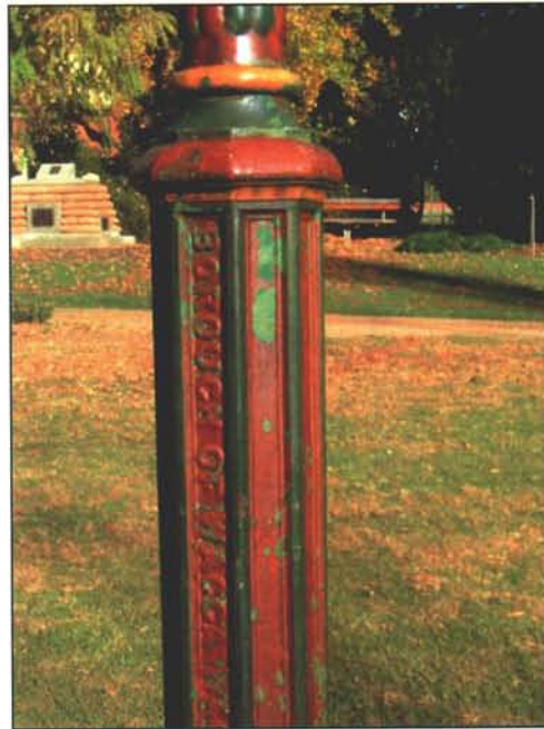
Type 1: - red green peeling paint
