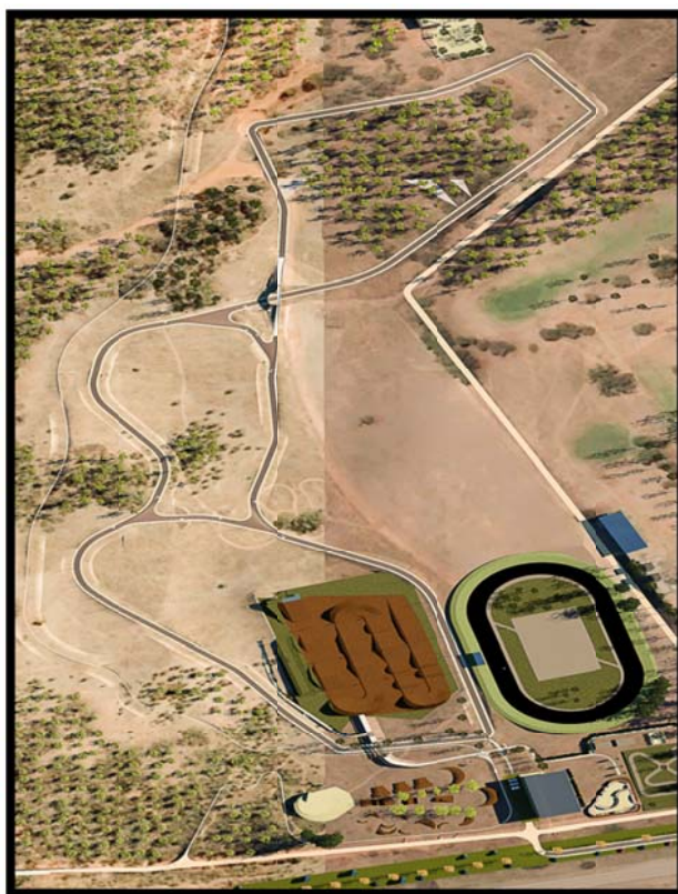
Figure 6.5: Aerial view of proposed Criterium Track at Pomingalarna Reserve.
