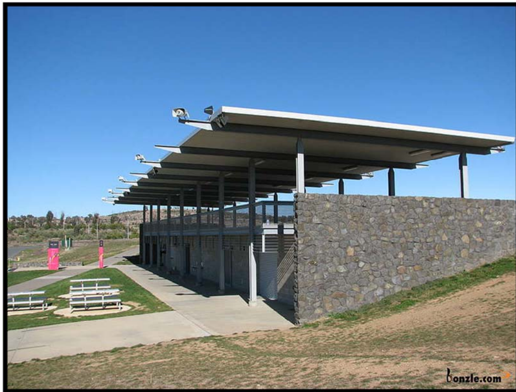
Figure 6.10: Amenities Building at Stromlo Forest Park, Canberra.
