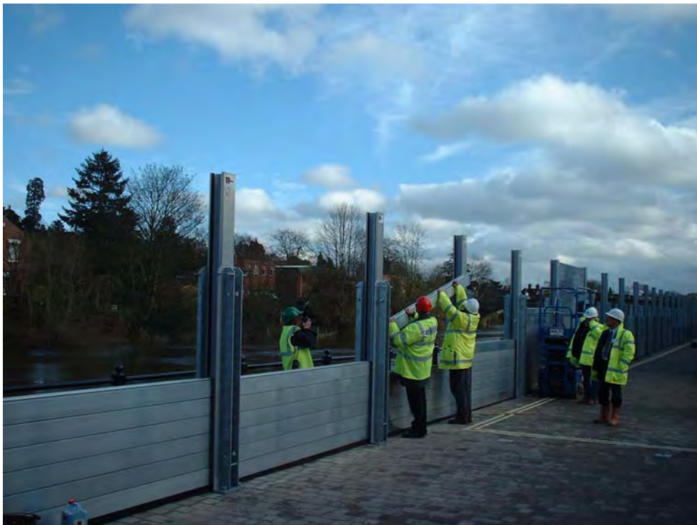
Bewdley Bridge, UK: Trial Installation of Bauer-IBS Demflood System
