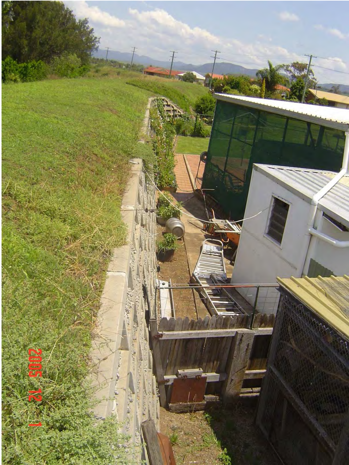
CRIB WALL LEVEE
