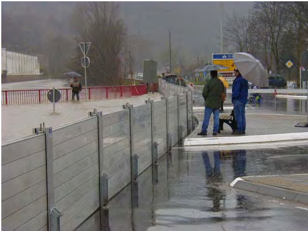
City of Alf, Germany: Barriers In use while flooding from the Mosel river
