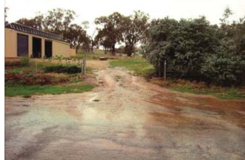
Plate 29 - Overland Flow in Argent Street (No Date) (Source: Bob Belling)
