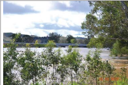
Plate 26 - Floodplain Between Sydney Street and Hume Highway (04/03/12 14:31) (Source: Matt Burgess)
