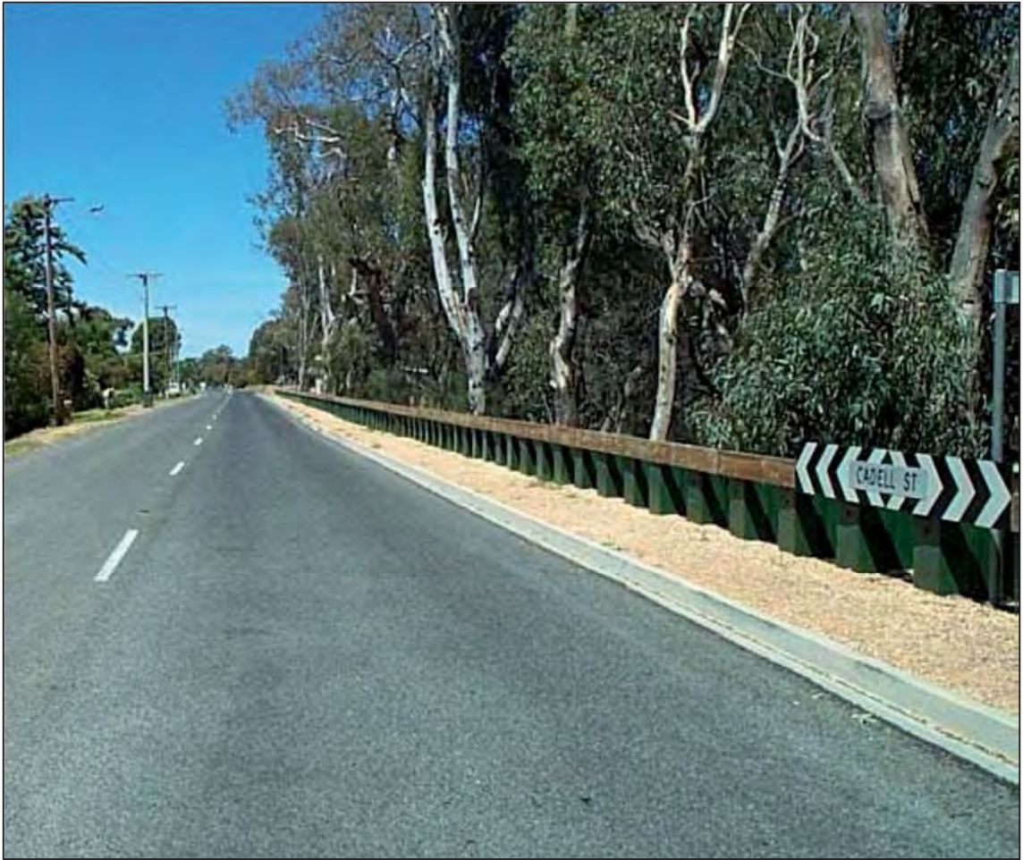
Sheet pile wall levee
