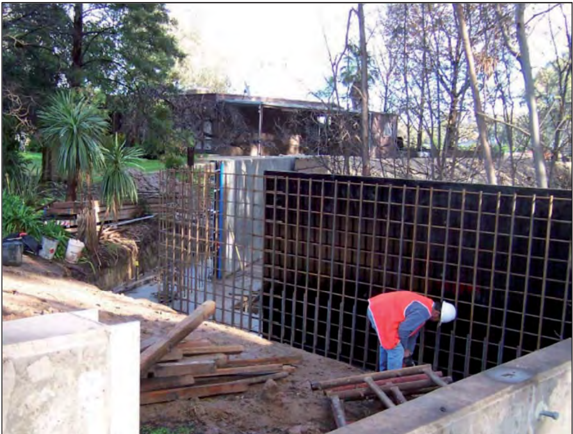
Cantilever wall levee
