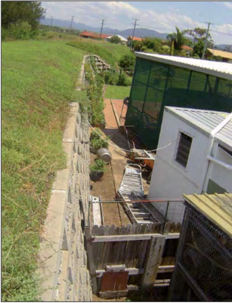
Hybrid crib-wall embankment levee
