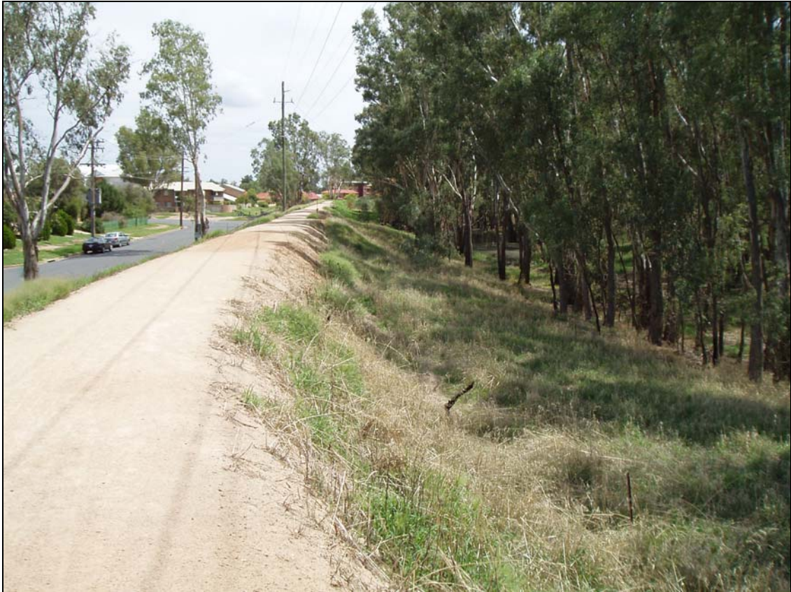
Plate 3: Levee bank adjoining residential development (Murrumbidgee River to the right)
