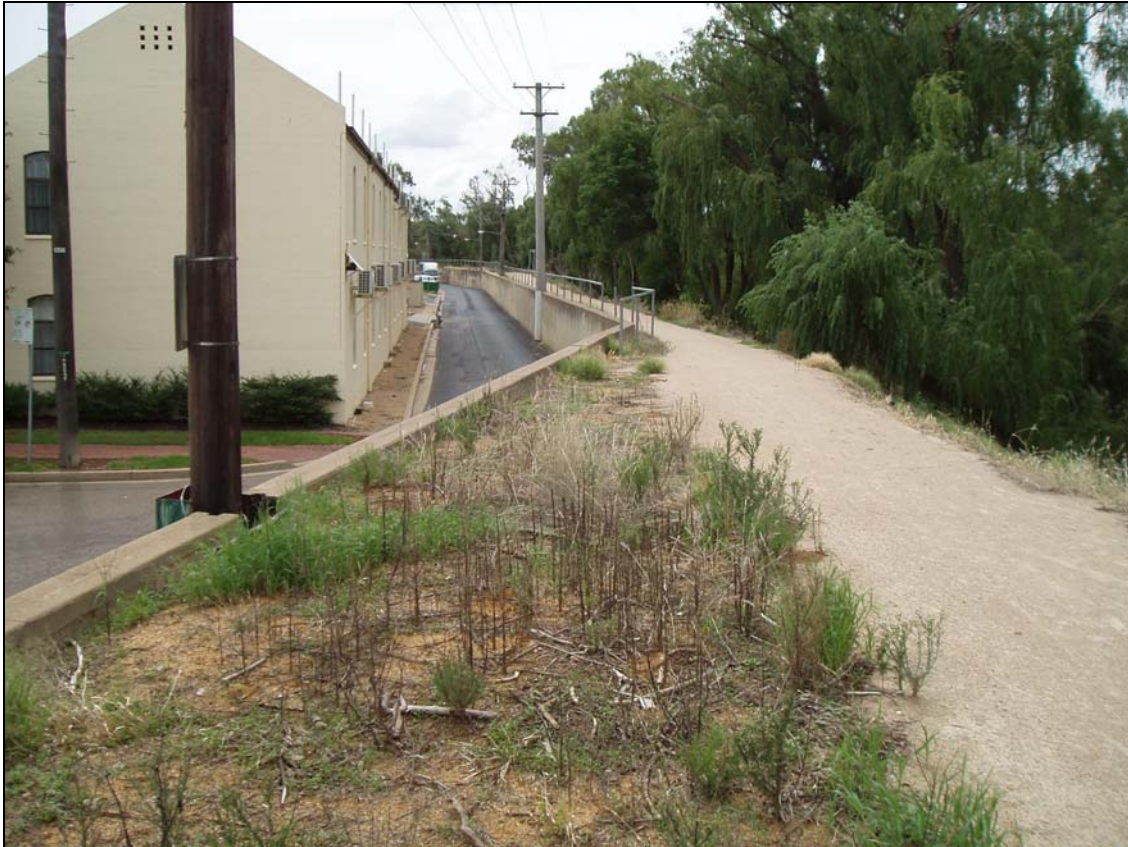
Plate 5: Levee bank at the rear of the Wagga Wagga CBD (note concrete retaining wall)
