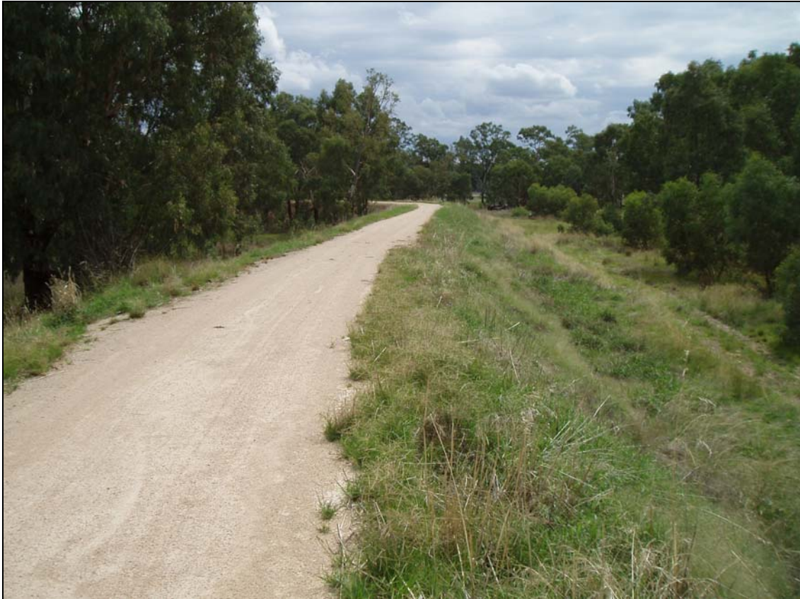
Plate 9: Main City Levee adjoining Flowerdale Lagoon (western section)
