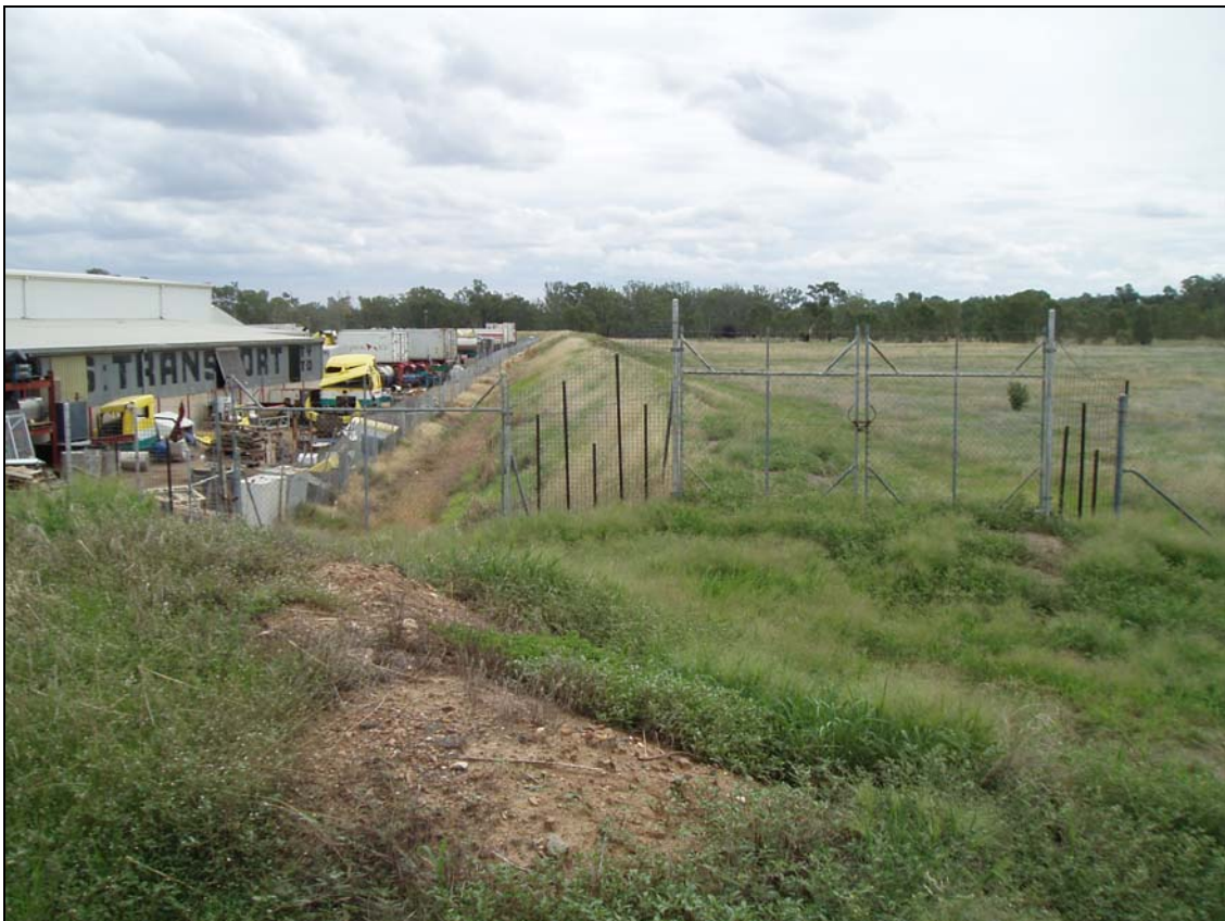
Plate 6: Northern section of Main City Levee
