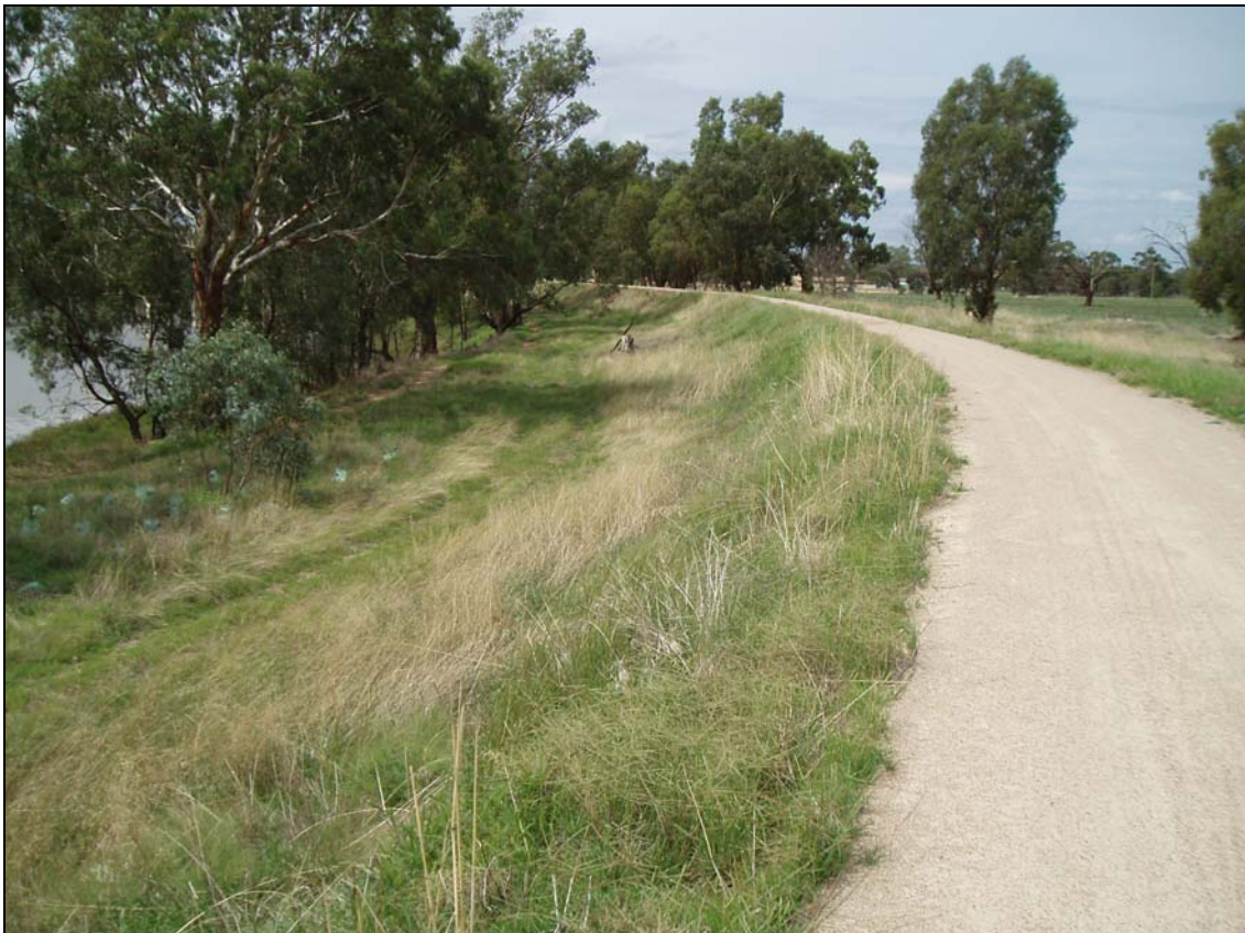
Plate 8: Main City Levee adjoining Flowerdale Lagoon (western section)
