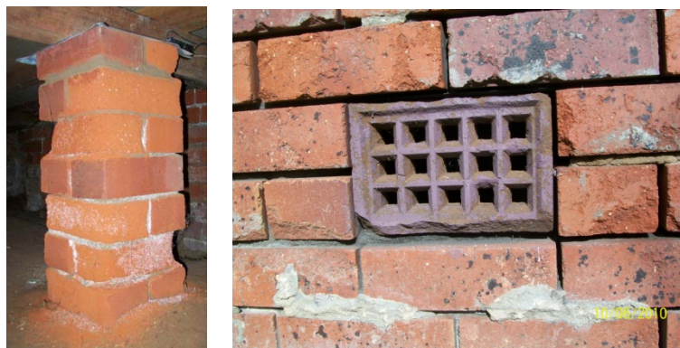
Figure 1: Salt damage to footings and mortar at a residential dwelling, Turvey Park, Wagga Wagga.
