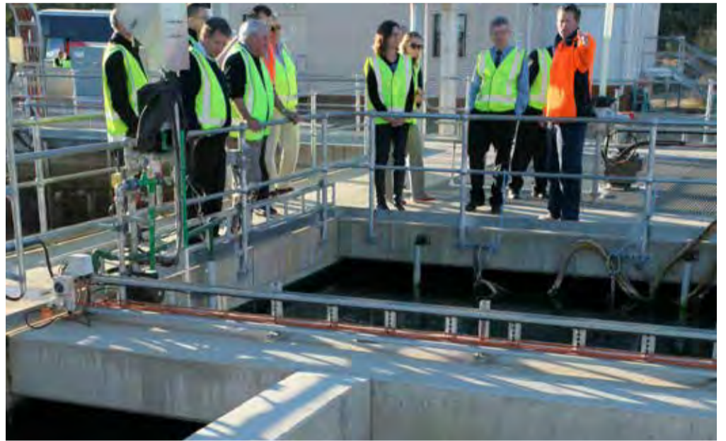
Above: Delegates from the LGSA Water Management Conference whilst on a site tour of The Narrung Street Sewage Treatment Plant.
