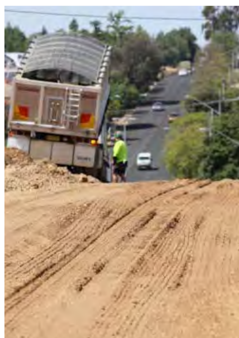
Above: Rehabilitation works underway in Mitchelmore Street, Wagga Wagga.
