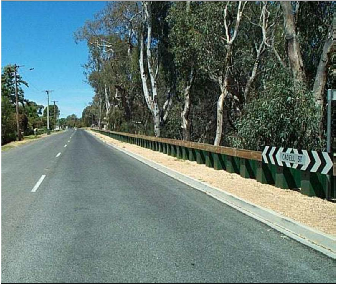
Sheet pile wall levee
