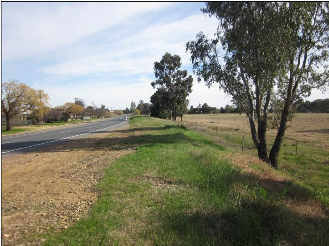
Figure 2.4: East Street (Bank Two) Levee - looking west along Mill Street, chainage 200
