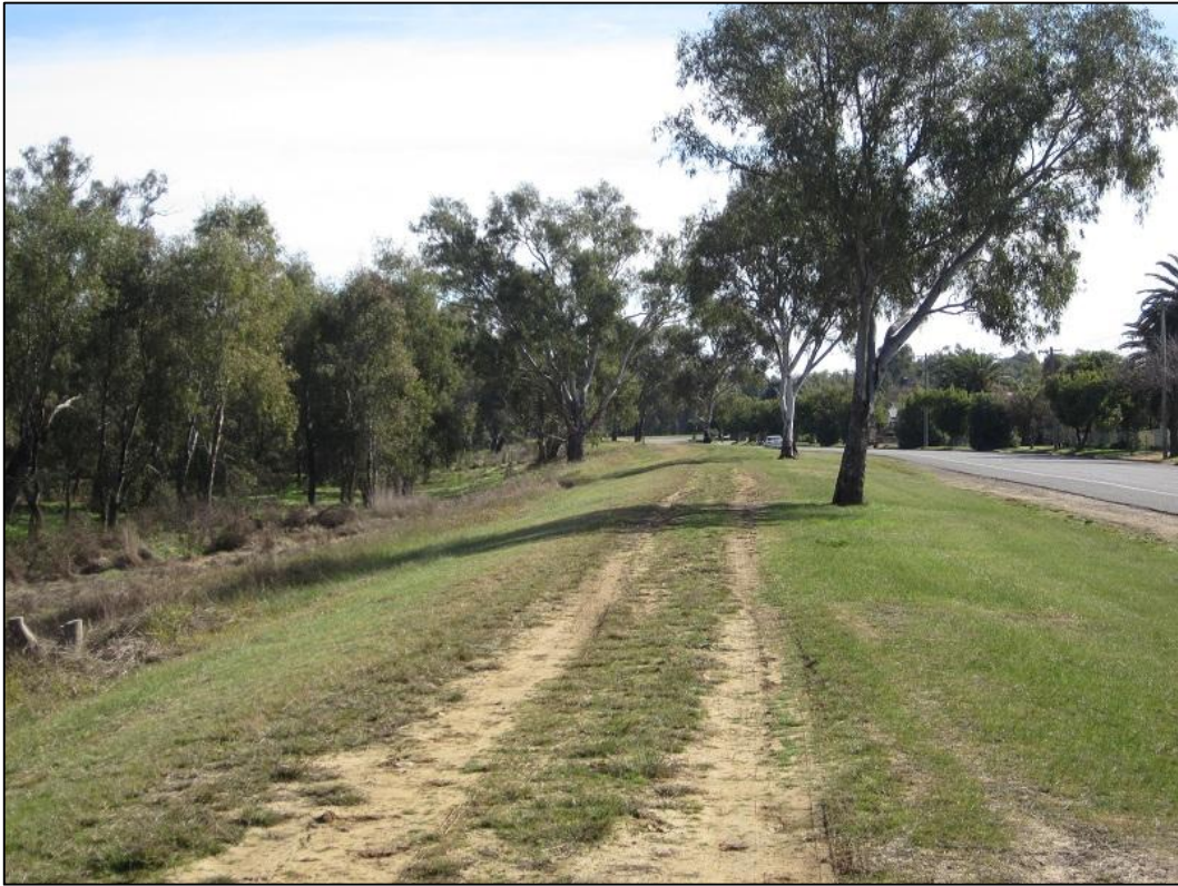
Figure 2.3: North Wagga Wagga Levee - looking north along Wall Street, chainage 4200
