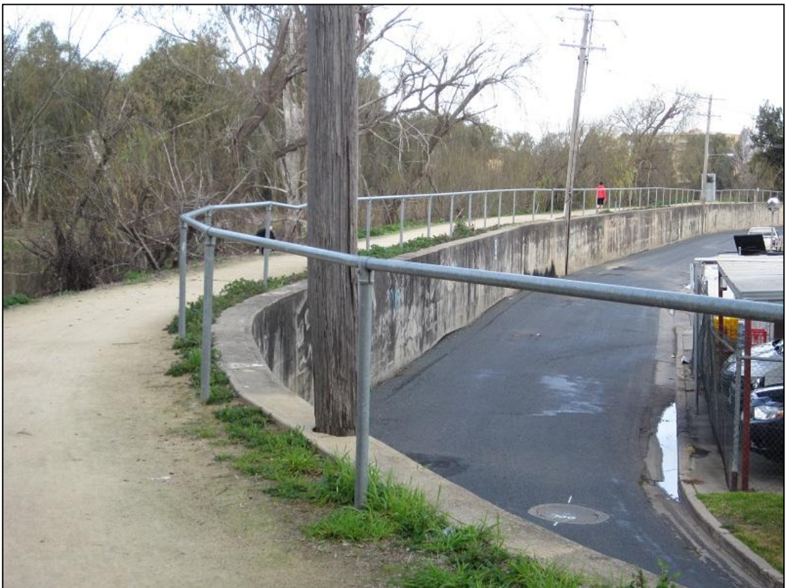
Figure 2.2: Main City Levee - concrete wall levee looking south along Cadell Place, chainage 4500
