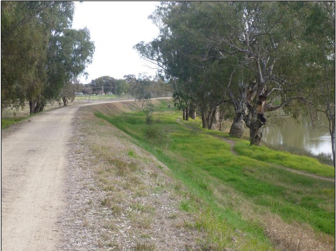
Figure 2.1: Main City Levee - embankment levee looking south near Flowerdale Lagoon, chainage 500
