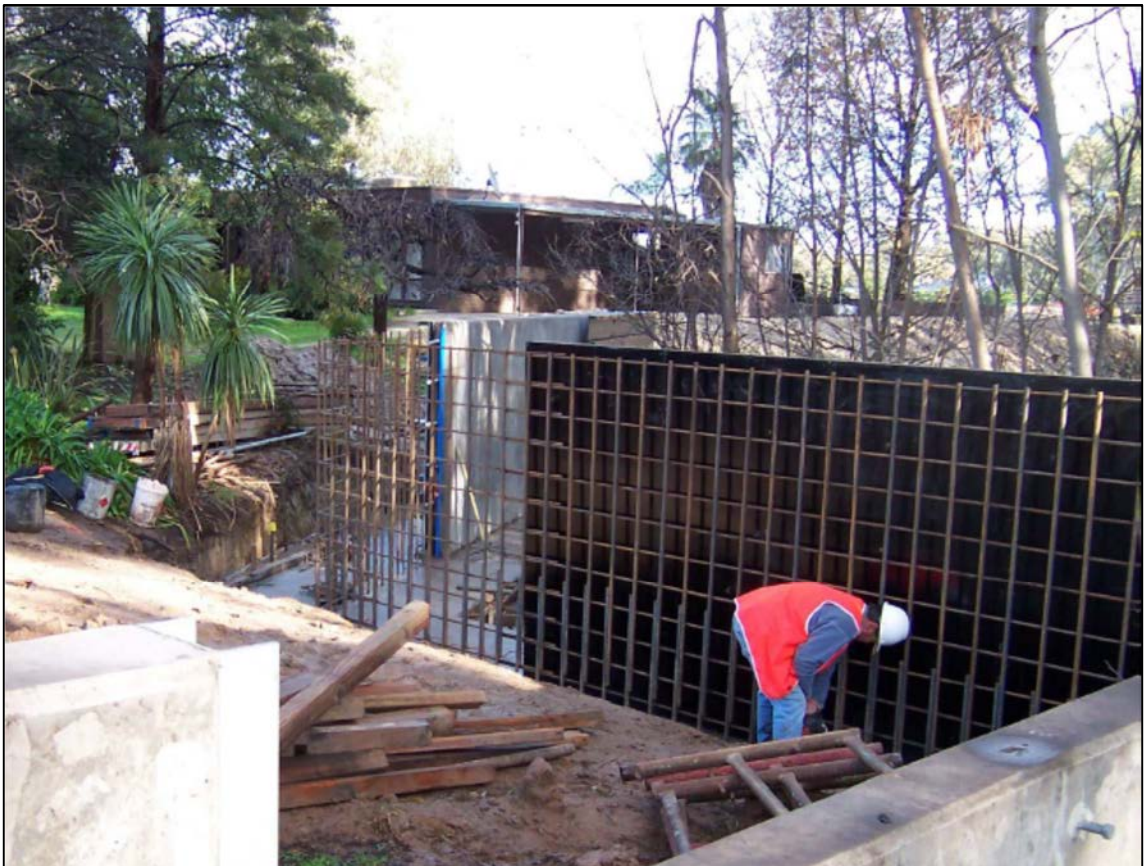
Cantilever wall levee
