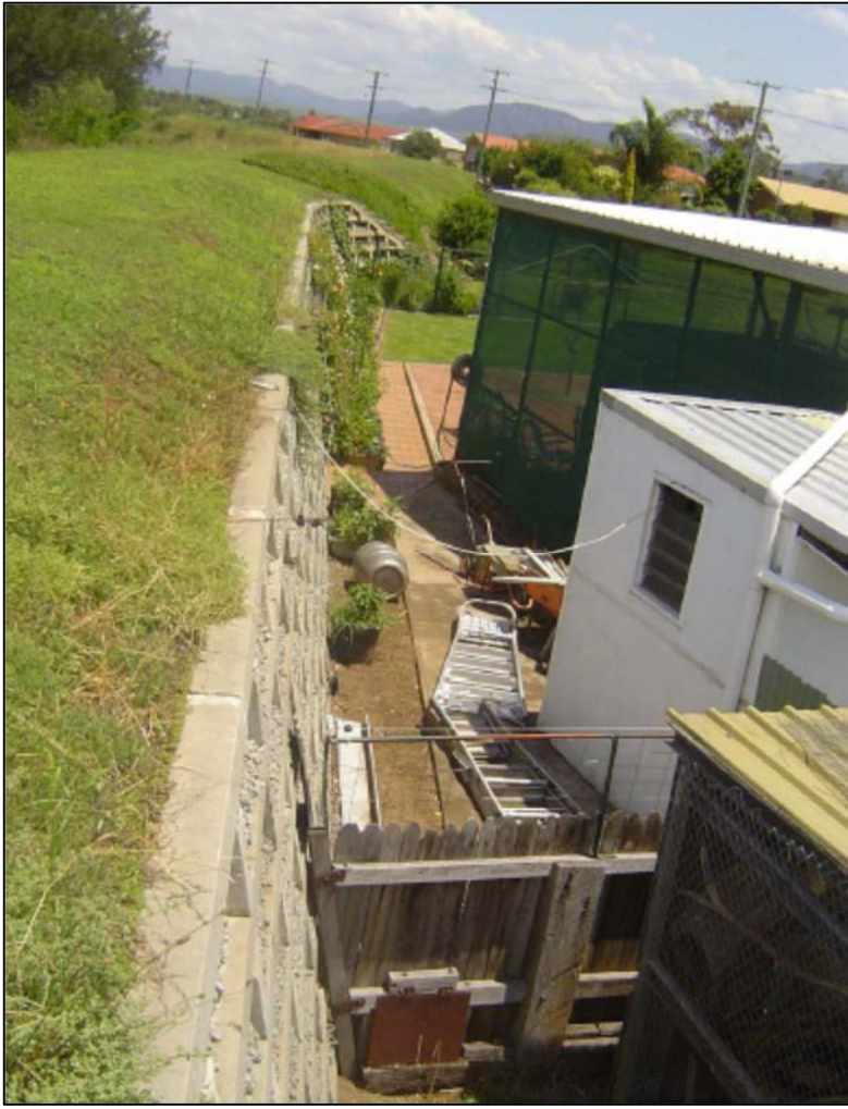
Hybrid crib-wall embankment levee
