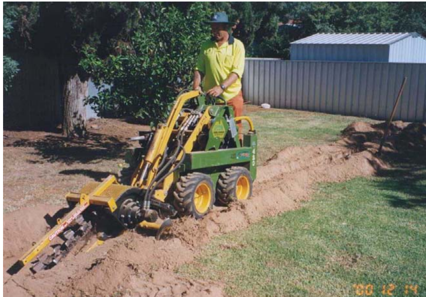
Installation of rear of block drainage
