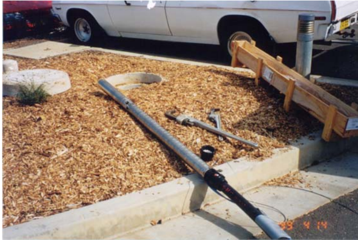
Typical bore being installed
