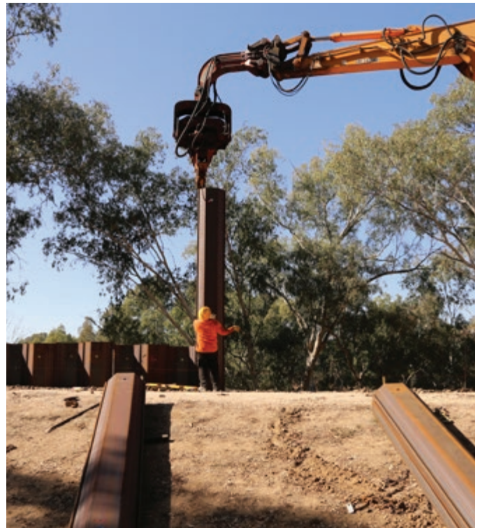
Capped sheet piles raise the height of the levee.
