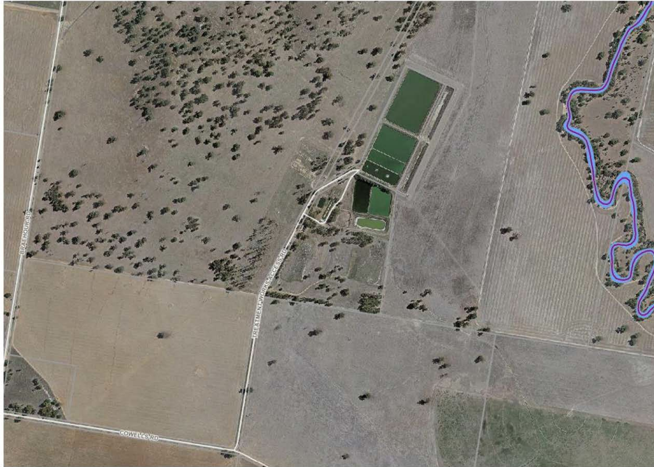
Forest Hill Sewage Treatment Plant
