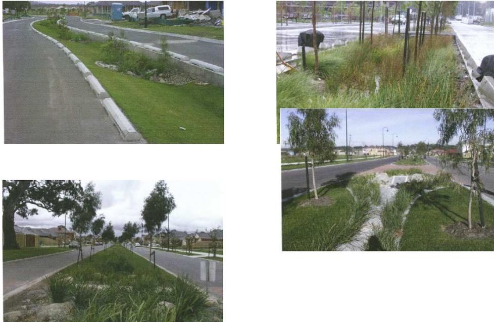
Figure D5.2 Typical bio-retention swales (Source: Melbourne Water)
