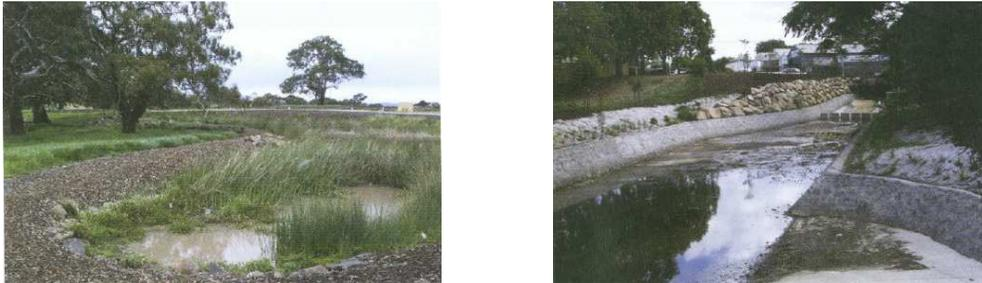
Figure D5.1 Typical sediment basins (Source: Melbourne Water)
