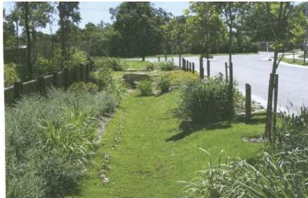
Figure D5.4 Swale and buffer system (Source: Melbourne Water)
