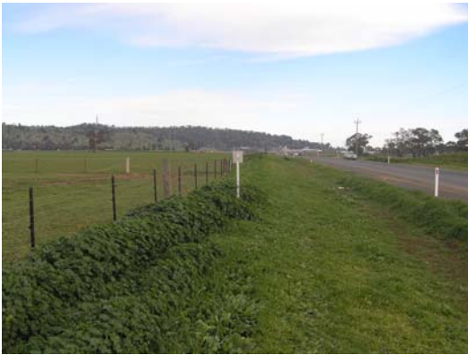
Photo 3.1: Table drain adjacent to Copland Rd
