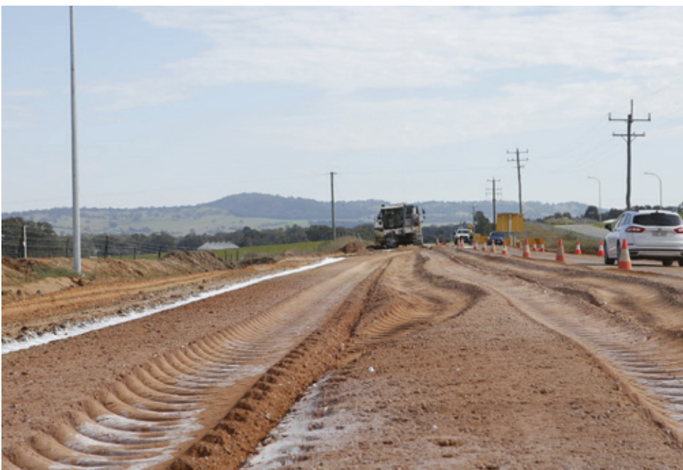
TAKING SHAPE: Lime stabilisation works on Old Narrandera Road as part of 2023 upgrade project.
