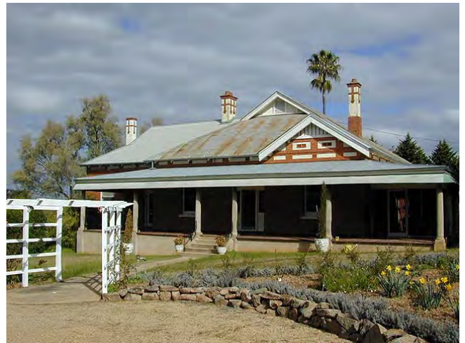
RMB 1011A Kooringal Road, former Kooringal Homestead
