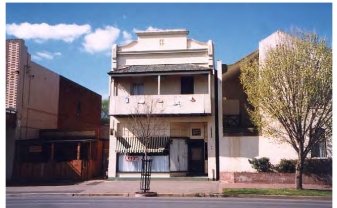
151 Fitzmaurice Street, one of the most intact shopfronts in Fitzmaurice Street and retaining its first floor balcony.
