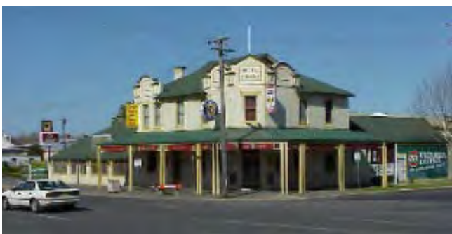
The former Bridge Hotel [to the left], many of Fitzmaurice Street's intersections are marked by hotels.
