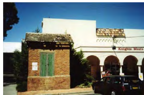
Electrical substation, near Knight's meats.
