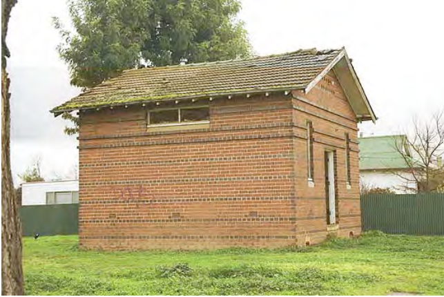
Electrical sub-station, cnr Crampton & Simmons Streets
