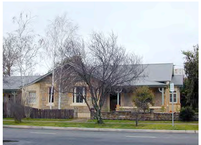
35 Dobbs Street, cnr Kincaid Street
