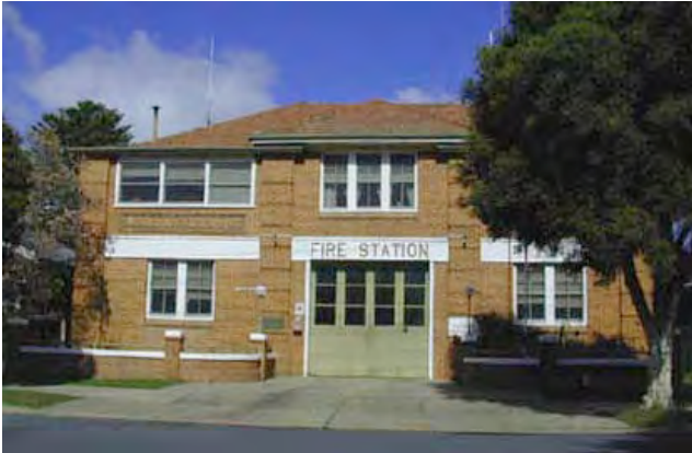
36 Morrow Street, Fire Station
