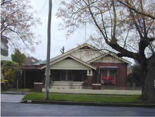
10 Trevor Street, typical of development in this street
