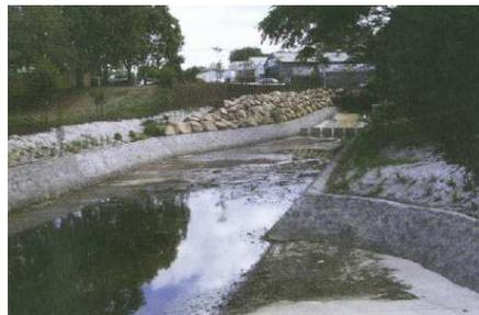
Figure D5.1 Typical sediment basins (Source: Melbourne Water)
