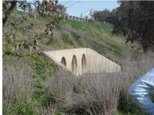
Photo 2.2: Culvert under Olympic Hwy
