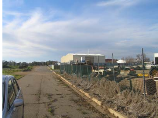
Photo 3.2 Kerb & Gutter in Tarcoola Rd
