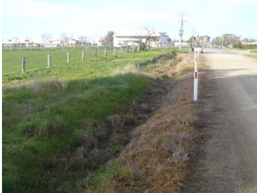
Photo 3.1 Table drain – eastern side of Koorungal Road
