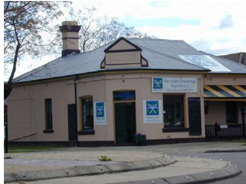
Front on view showing the two street elevations and the attached residence.
