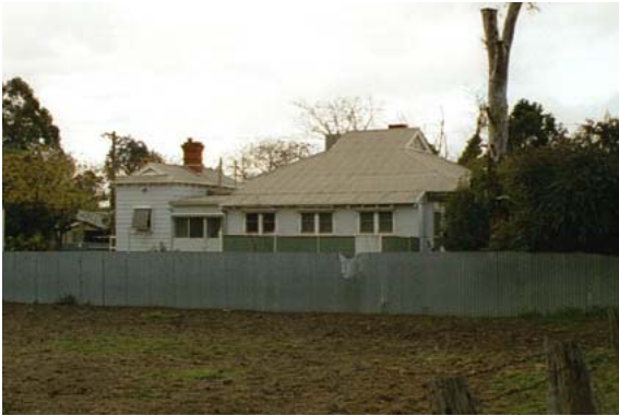
Side view showing former lock-up to the rear of the building
