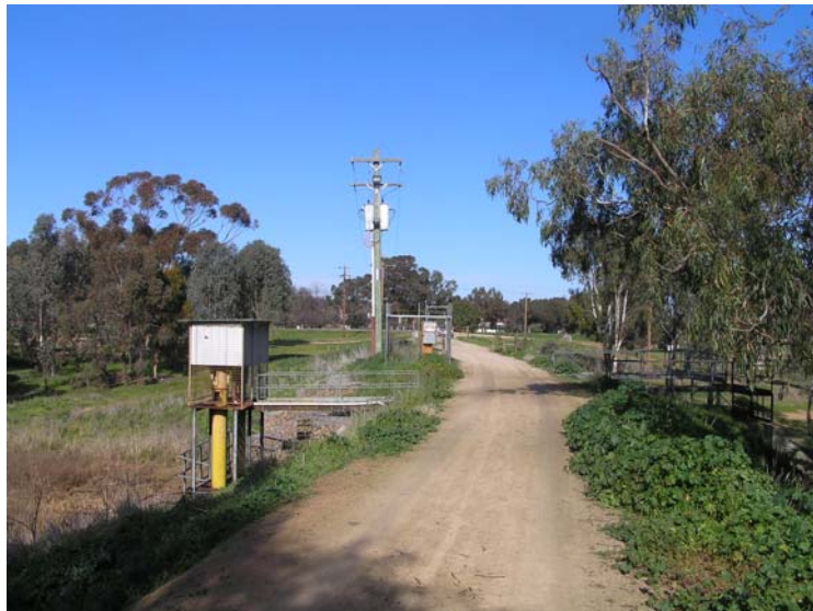
Photo 4.1: Top of Levy and Pumps
