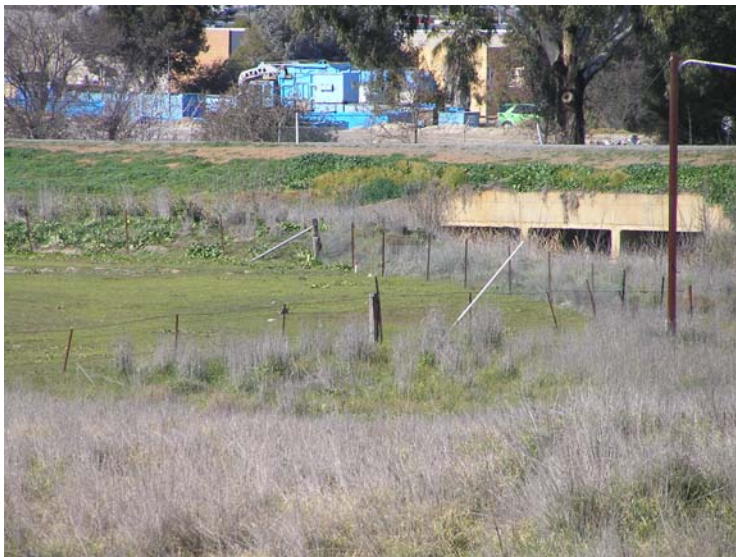
Photo 3.1: Glenfield Carrier – culvert under Sturt Hwy
