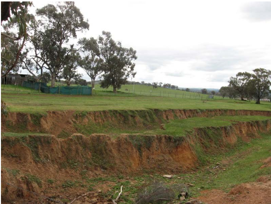
Plate 4. Looking south from a vehicle track, showing the effect on the drainage line of concrete stream channelling beneath the vehicle overpass, Lloyd study area.
