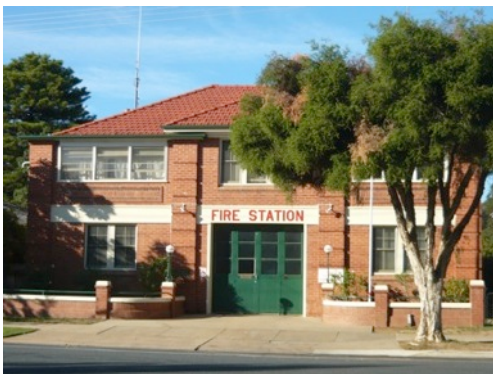
Figure 5.3. Fire Station (K Beasley 2013)
