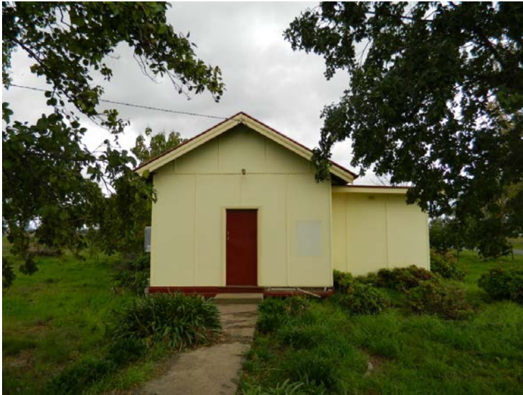
Figure 4.34. The basic fibro building that was once the church at Gumly Gumly, now used as a small community hall building (G Shaw 2012).
