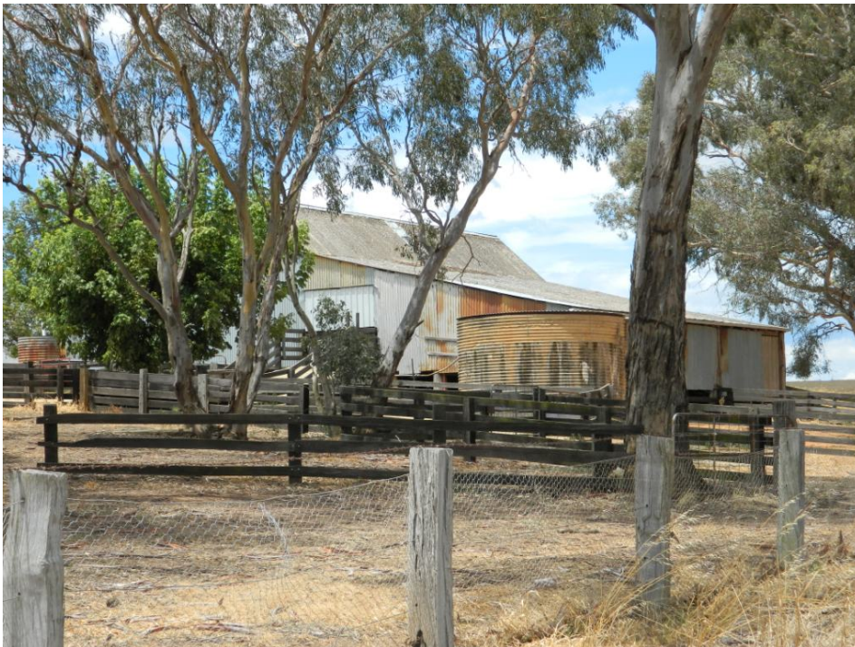
Figure 4.23. Woolshed at Cressy Farm at Pulletop (G Shaw 2012)
