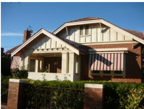
Figure 5.4. Residence at 62 Tompson Street (K Beasley 2013)
