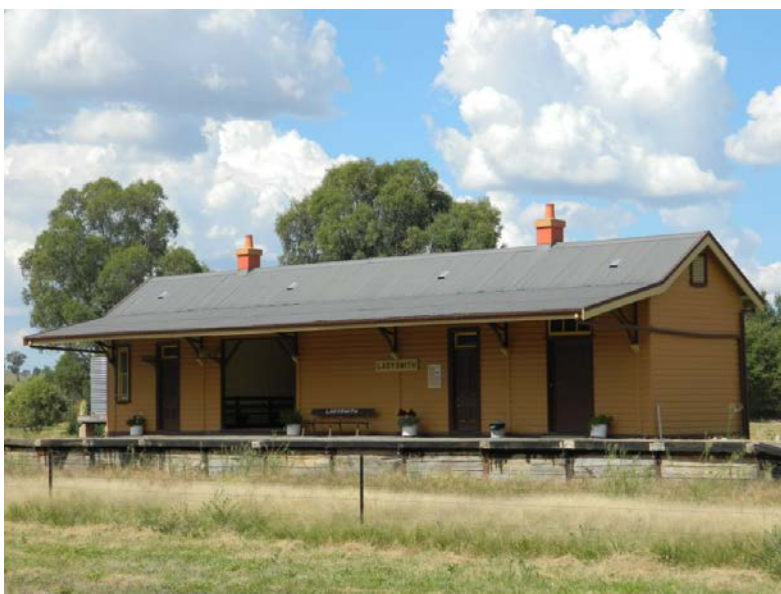
Figure 4.41. The main platform at Ladysmith Station now part of a railway museum (G Shaw 2012).
