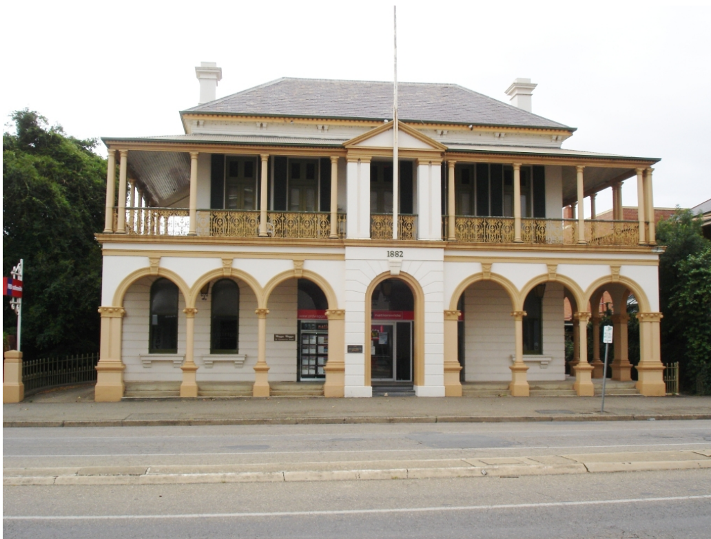
Figure 4.1. Former CBC Bank at 53-55 Fitzmaurice Street (N Thomson 2012).
