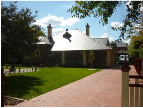
Figure 5.7. Residence at 87 Tompson Street (K Beasley 2013)
