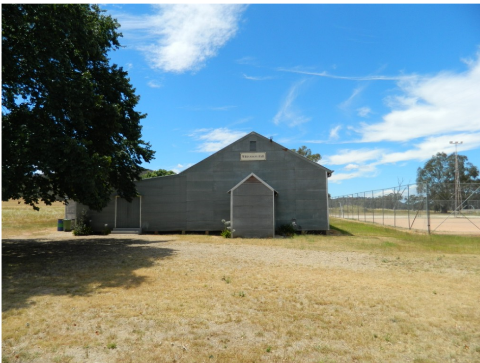
Figure 4.37. The Burrandana Hall and tennis courts remain well utilised by the local community (G Shaw 2012).
