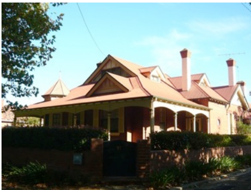
Figure 5.6. Residence at 97 Gurwood Street (K Beasley 2013)
