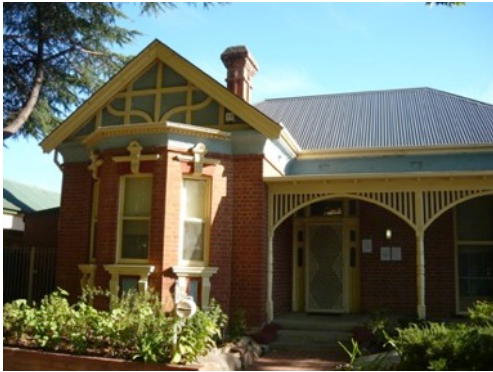
Figure 5.5. Residence at 53 Gurwood Street (K Beasley 2013)
