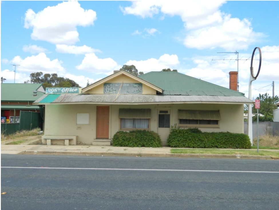
Figure 4.11. The former Uranquinty store that has now been relocated to the neighbouring modern store within the service station (G Shaw 2012).
