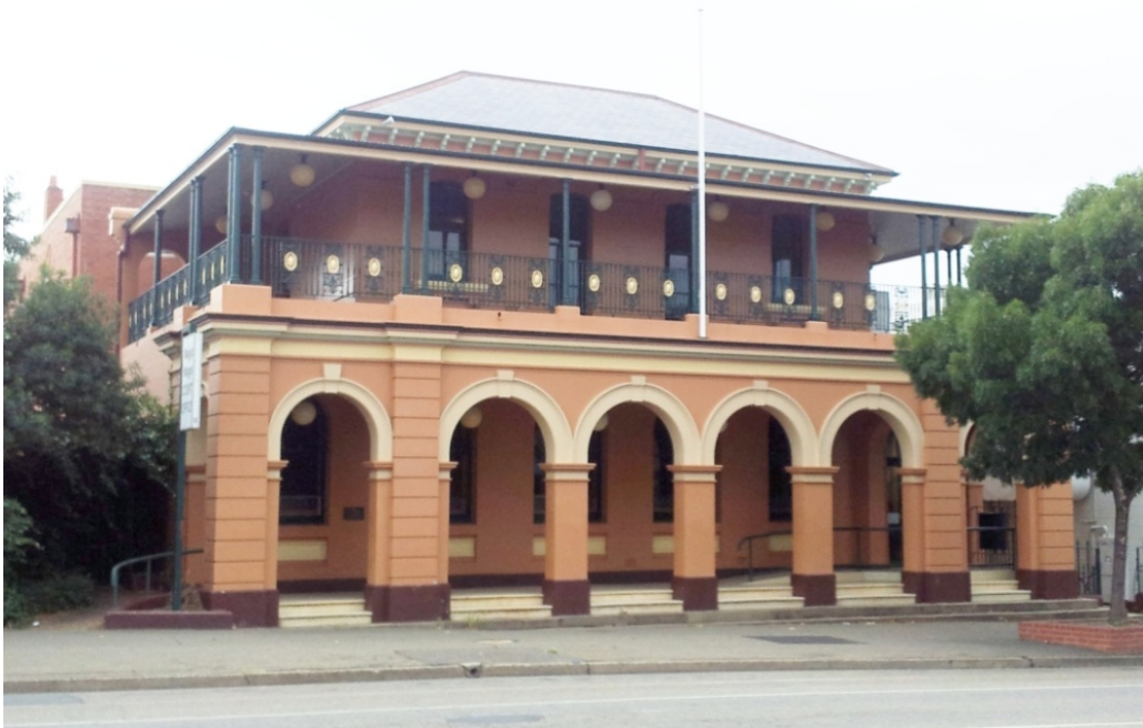
Figure 4.3. The former Post Office at 49-51 Fitzmaurice Street (N Thomson 2012)
