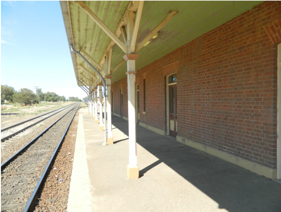
Figure 4.42. The Bomen Railway Station that has recently been subject to rehabilitation works to the main building (G Shaw 2012).
