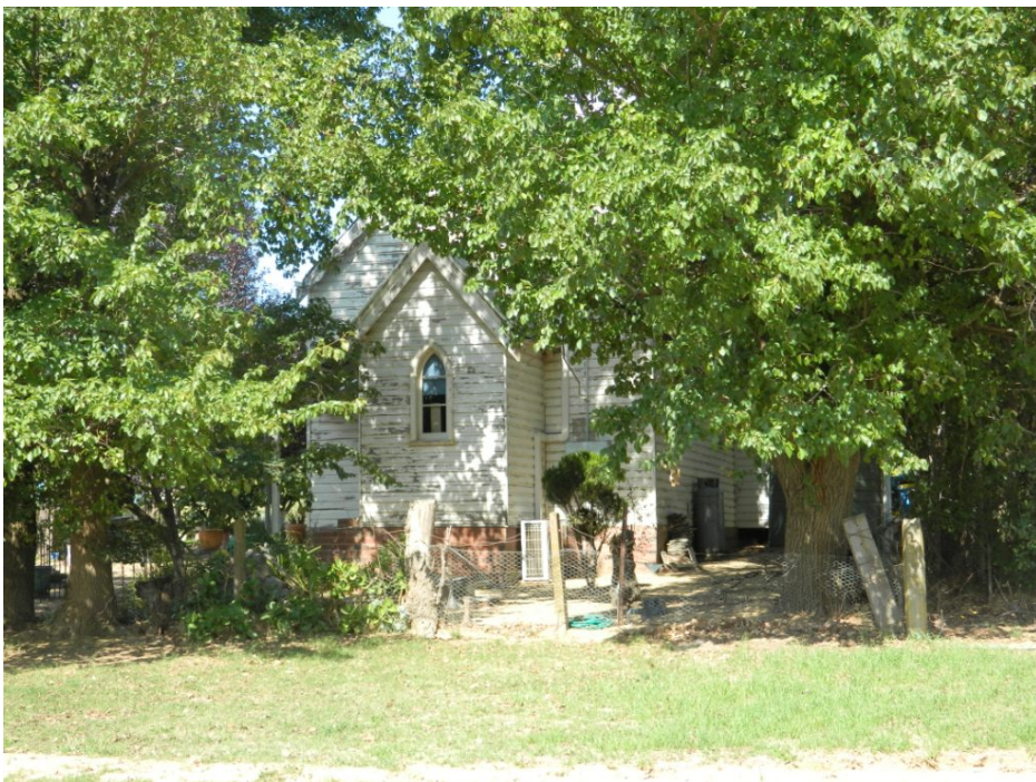
Figure 4.33. Former Methodist church at Ladysmith, now a private residence (G Shaw 2012).
