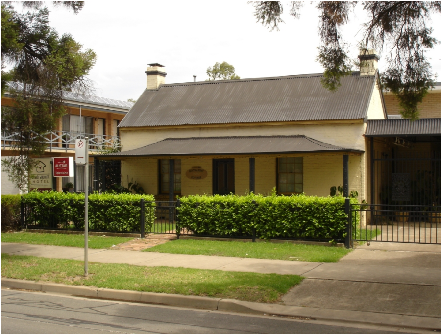
Figure 4.14. Cottage on Tarcutta Street now an office for a motel (G Shaw 2012).
