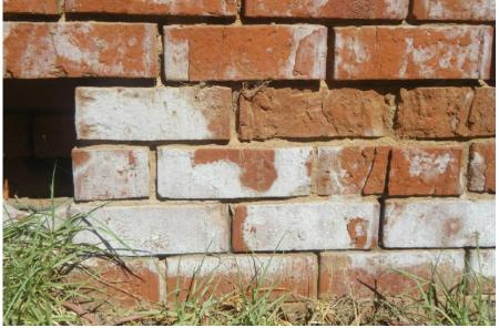
Figure 3 – Impacts of salinity on brickwork
