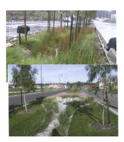
Figure D5.2 Typical bio-retention swales (Source: Melbourne Water)
