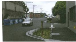
Figure D5.3 Typical bio-retention basins (Source: Melbourne Water)
