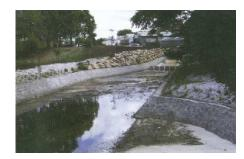
Figure D5.1 Typical sediment basins (Source: Melbourne Water)
