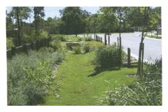
Figure D5.4 Swale and buffer system (Source: Melbourne Water)
