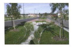
Figure D5.2 Typical bio-retention swales (Source: Melbourne Water)
