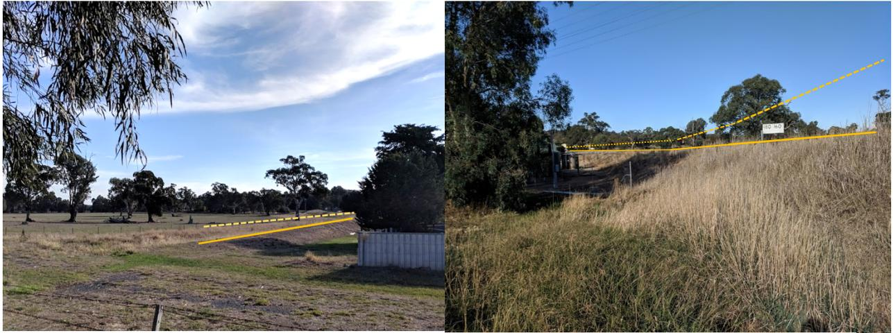
East end (left) and west end (right) of levee with crest in yellow and approximate additional height in yellow
